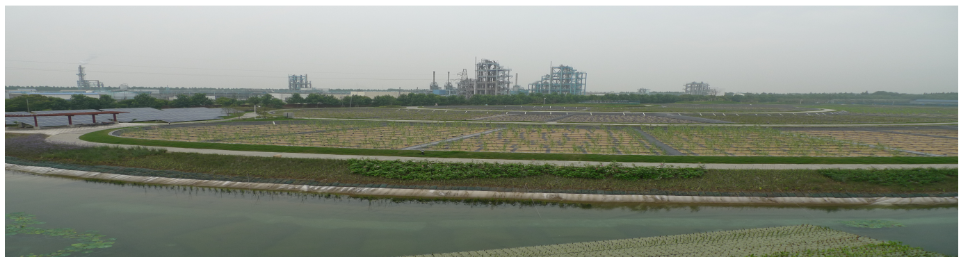
Vertical subsurface flow constructed wetland
